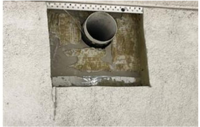
Phase 1 South Elevation
